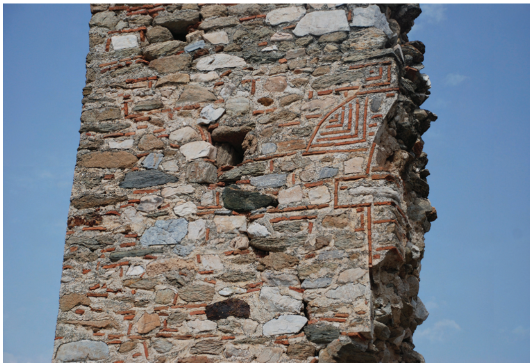
Plate 52. Servia. Tower of the citadel, masonry detail. (Photo: Flora Karagianni)
